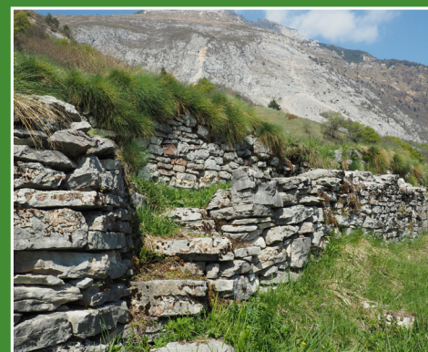
Muri a secco / Dry stone walls
